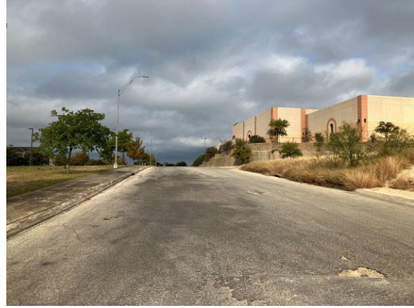
Cinema Ridge at Subject Facing Northwest
