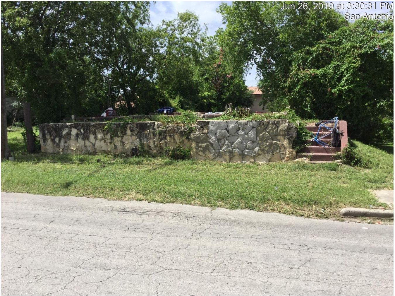
Concrete to be removed
