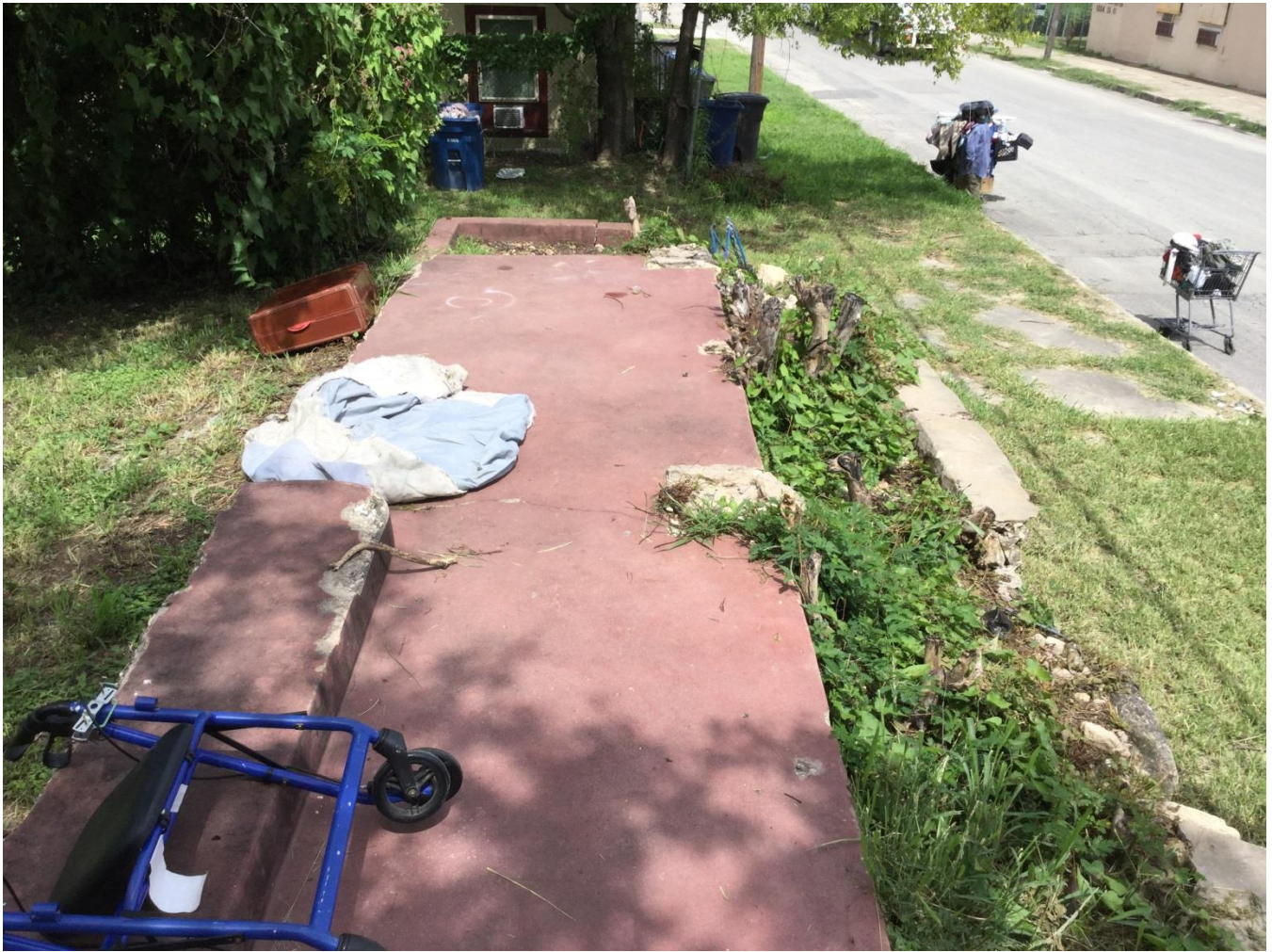
Concrete to be removed
