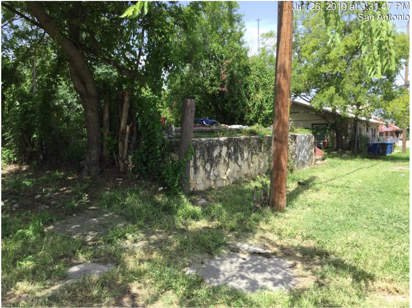
Concrete to be removed
