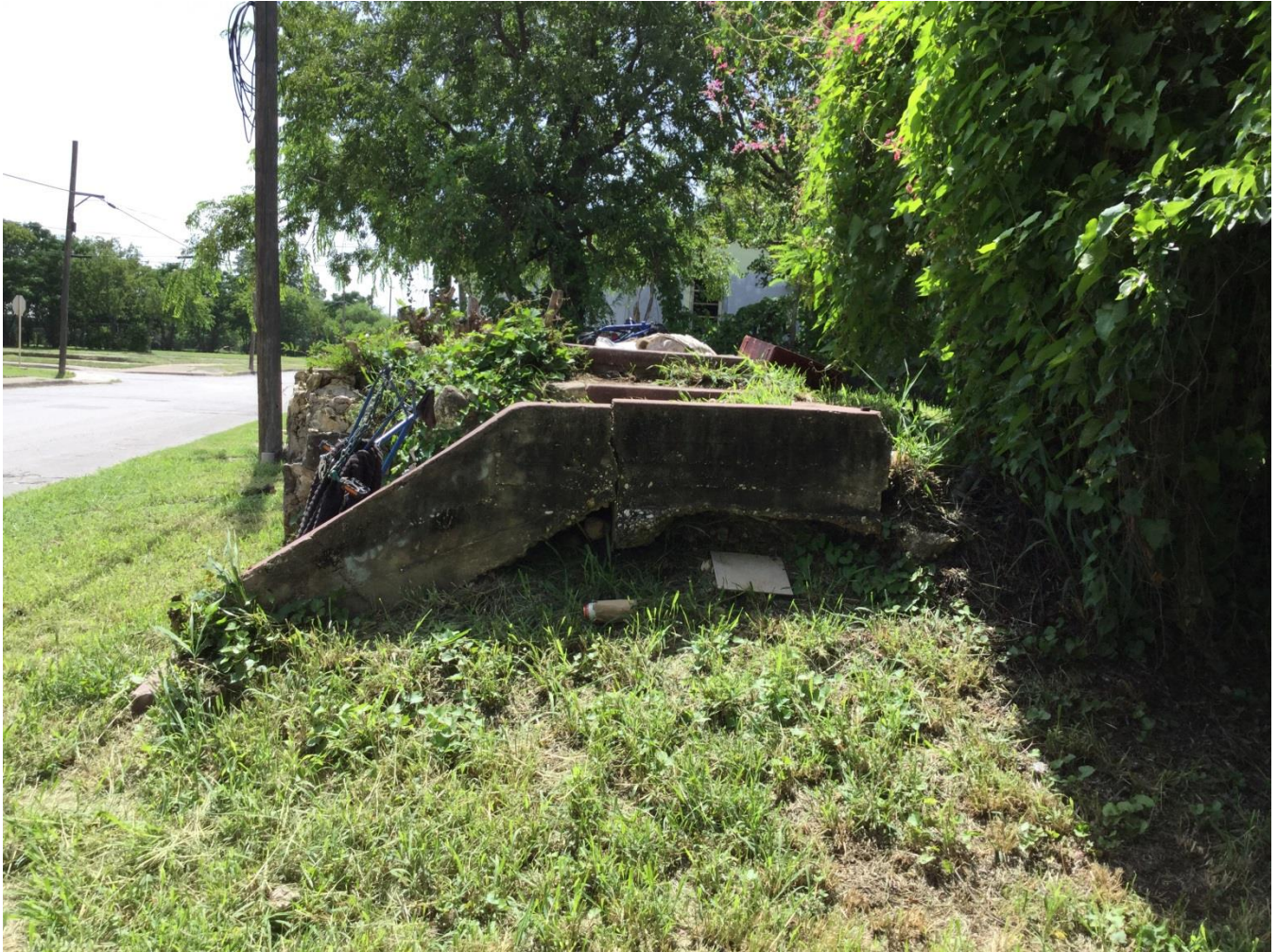
Concrete to be removed
