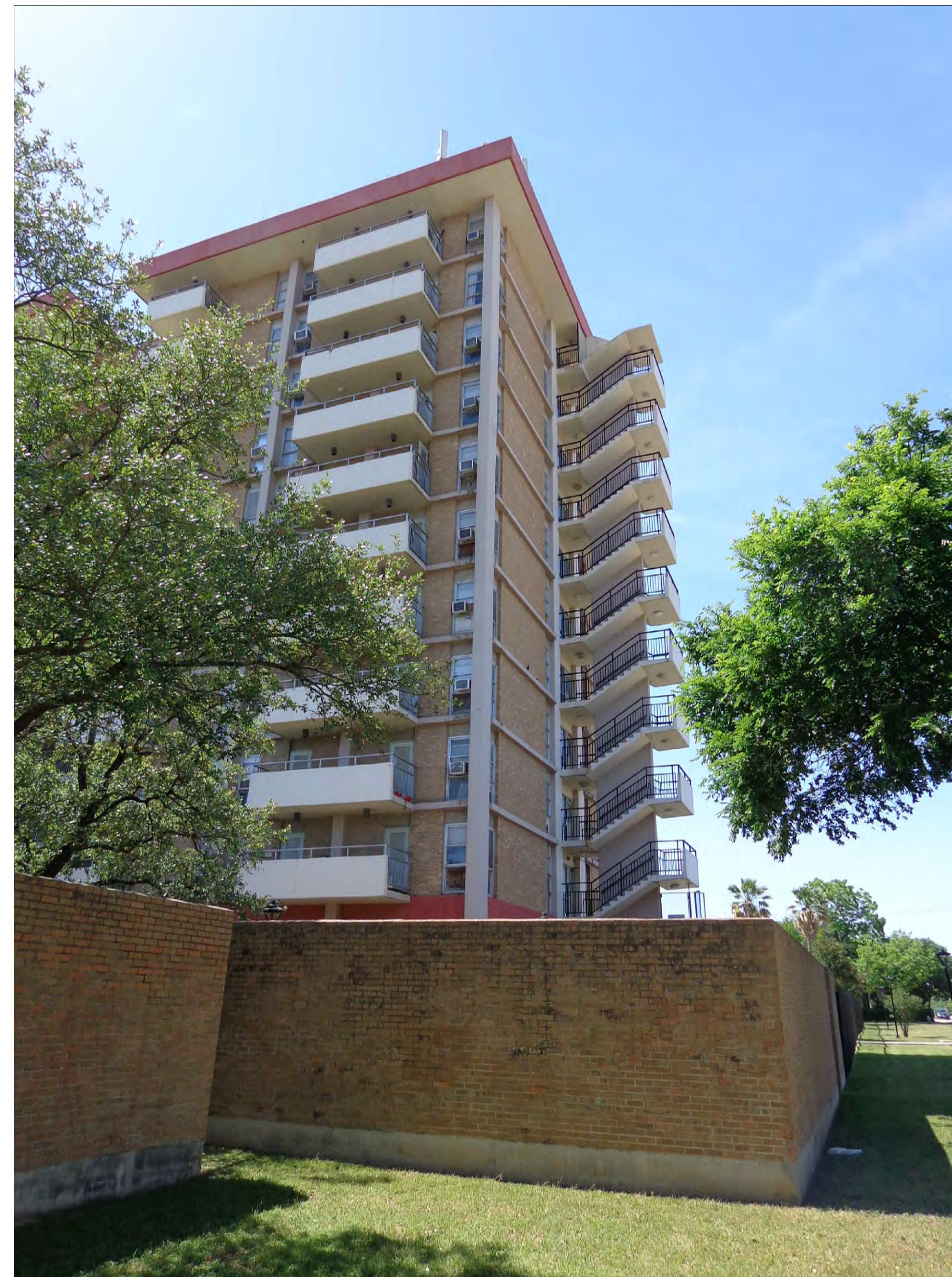
2 SOUTH ELEVATION PHOTO NTS
