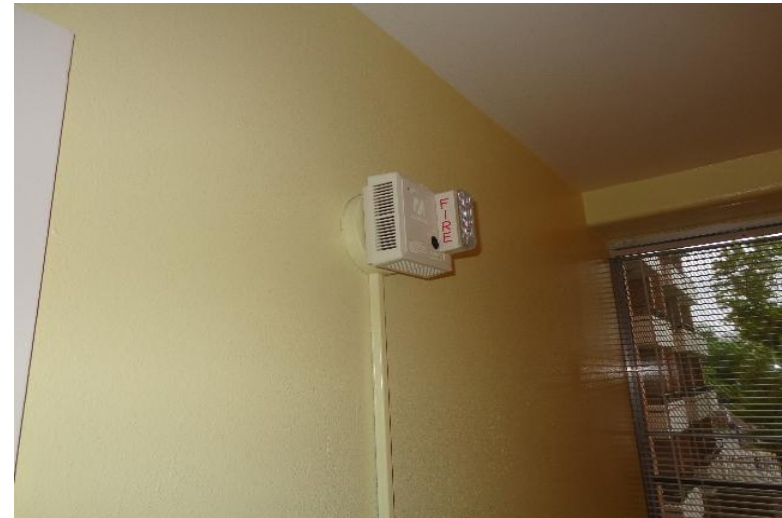
Photo #4 Smoke alarm strobe to be marked for removal by appropriate personnel.
